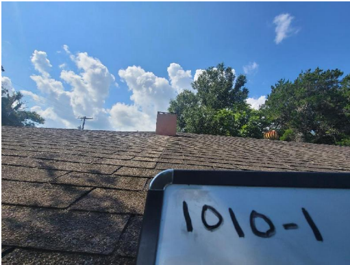
1010-1 Asphalt Shingle/Tar Typical Exterior Roof
