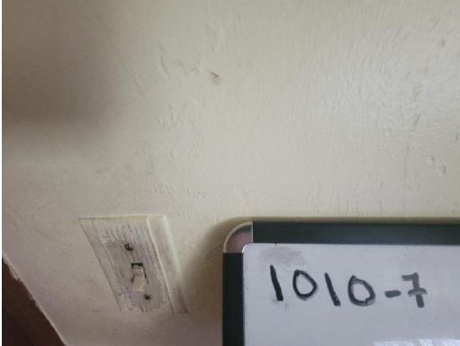
1010-7 Plaster/Skim Coat/Rough Coat Typical Interior Walls/Ceilings
